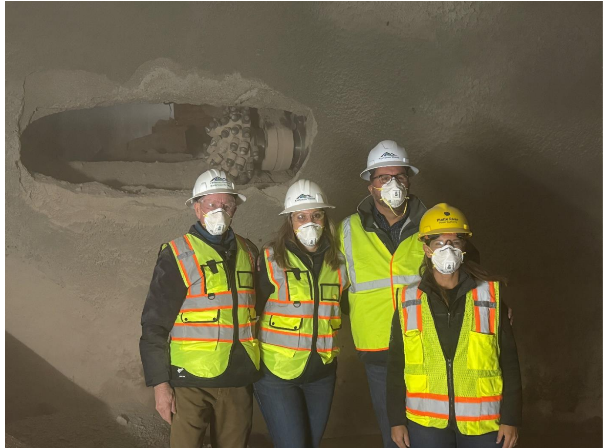
A roadheader was used to hole through and connect the upstream and downstream tunnel sections.
