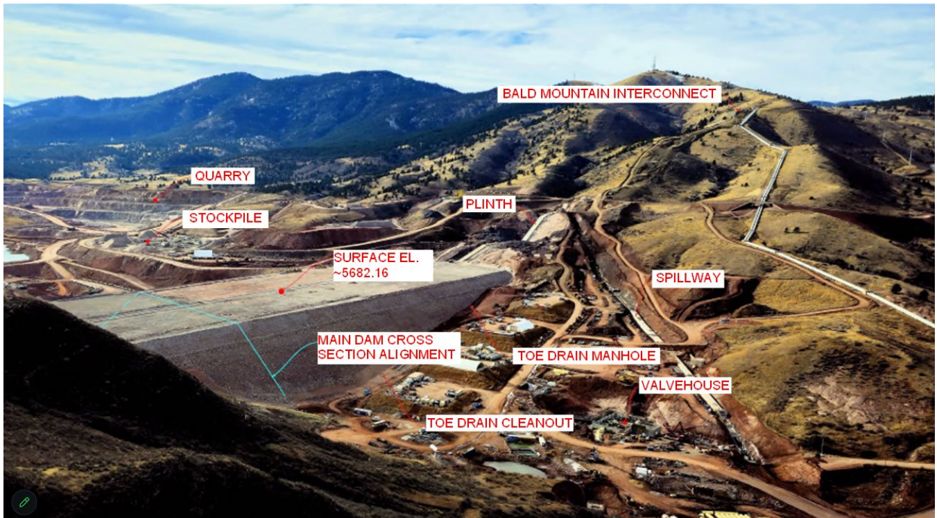
Chimney Hollow reservoir main dam construction (looking southwest)
