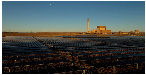
Rawhide Prairie Solar located at Rawhide Energy Station
