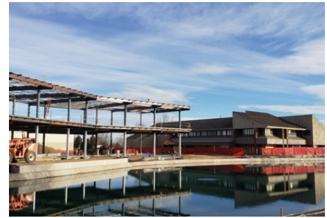
Construction of the new Platte River headquarters campus.
